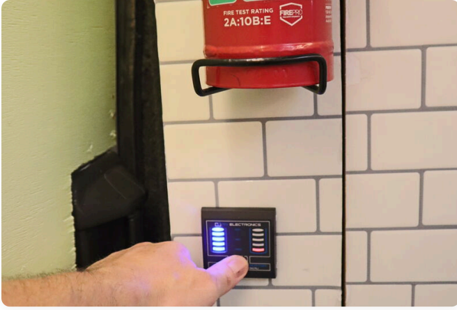
Water level gauge and the storage area built around the tank
