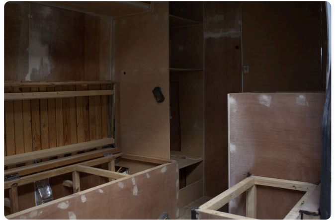
The whole interior filled, sanded and ready for paint
