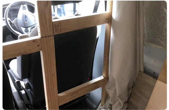
Building the insulated cockpit dividing wall — using reclaimed wood from the original panels
