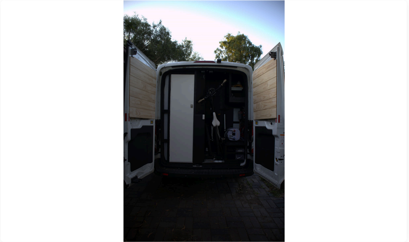
The finished garage — all electrical gear centralised in one ventilated area
